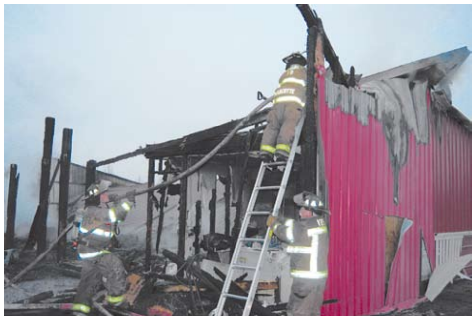
Photo courtesy VBT Fire Department
