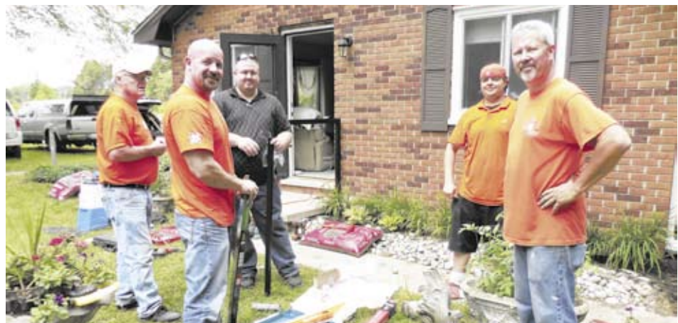
Team Depot volunteers working at the front of the Hanes home on Fret Road last Thursday were, from left: Len Harrington, Steve Larkins, Rob Lancioni, Mike Cooley, and Team Captain Brian Fitzgerald.
