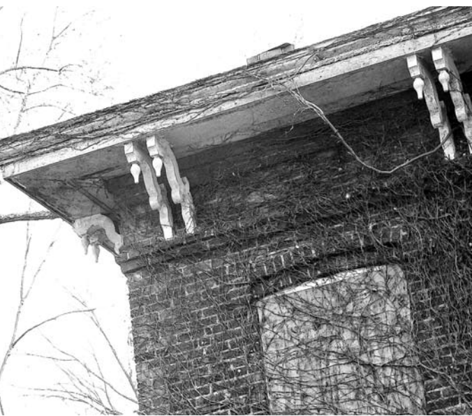
Photo by Samantha Luke, age 10 The Riggs house, built in 1867 at the corner of East Huron River Drive and Martinsville Road in the Riggs Heritage Park, is being demolished by Van Buren Township Board of Trustees. Budding photographer Samantha Luke took pictures of the corbels on the house and the Belleville Area Museum is asking the township to save the corbels. A few years back the township put a new roof on the house with the plan to restore the building, but left it to deteriorate instead.
