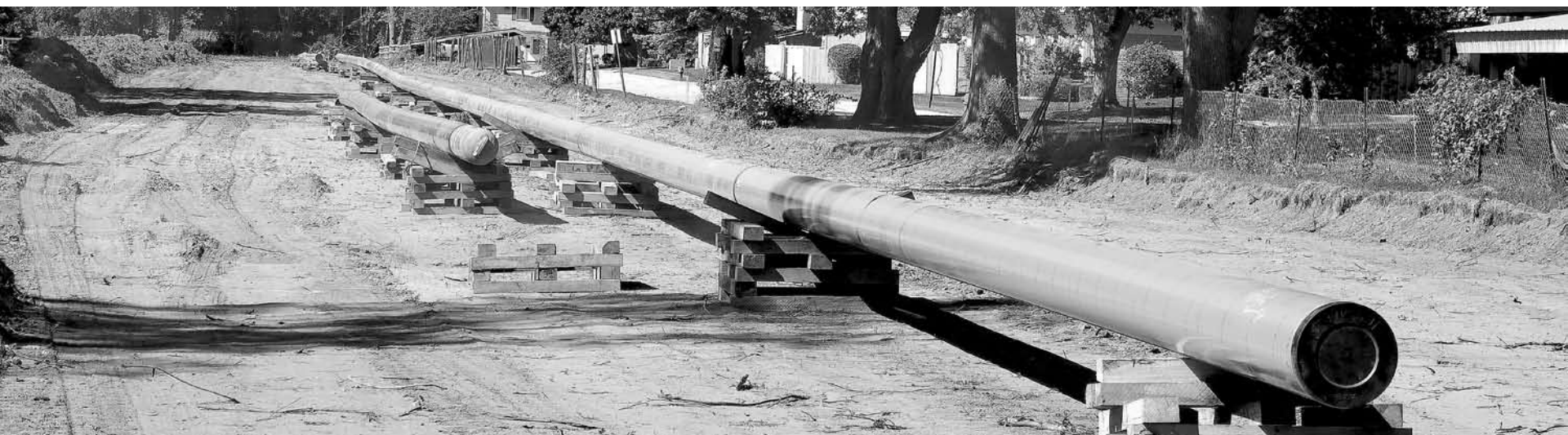
This 16" diameter pipeline being buried in the right of way next to a buried 1953 pipeline was seen Sunday west of Haggerty Road, near Robson. It is part of the Wolverine Pipeline that carries gas and fuel oil from Chicago to Detroit. Thirty-five new miles of pipeline now are being installed between Freedom Township in Washtenaw County and Romulus, where it will connect to an existing pipeline. The new pipeline goes right through Van Buren Township from Rawsonville Road on the west to Hannan Road on the east.
